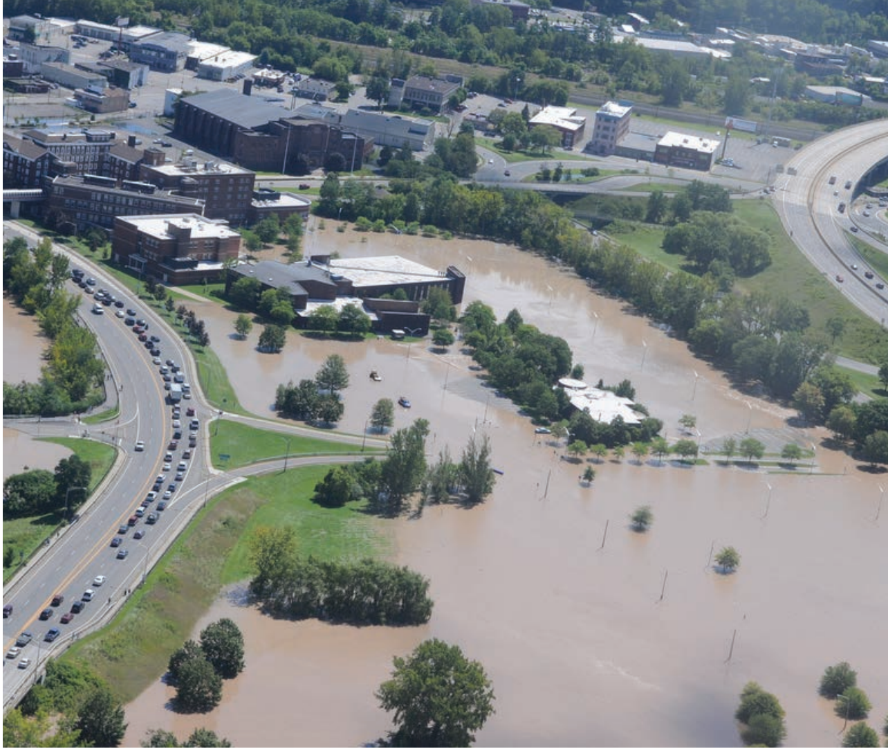
Schoharie County flood damage from Hurricane Irene.
